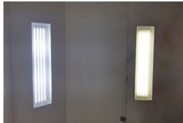
LED T8 bulbs (left) compared to old Fluorescent T8 bulbs (right) in a body shop
