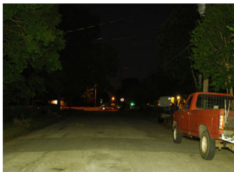
The same street illuminated by the LEDERL-20; an unquestionable difference. This LED light is designed as a flood to illuminate an area closer to the fixture.
