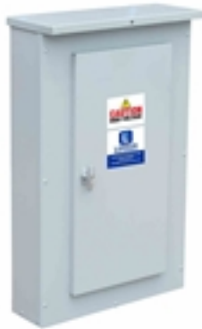
Image: MPD-PNL-3P-MCB-100A-208Y.120V-16.B-N3R
