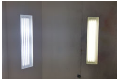
LED T8 bulbs (left) compared to old Fluorescent T8 bulbs (right) in a body shop
