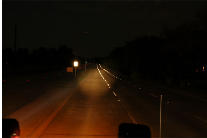
GL-2067 Illuminating a stretch of road about 5000 feet in length.
