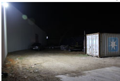
WAL-QP8- WP60PM-GRC50 LED light head mounted 15' high illuminating a 30' long by 50' wide parking area. Click Photo to Enlarge
