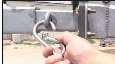
3. Remove the retaining pin from the base of the mast and set aside.
