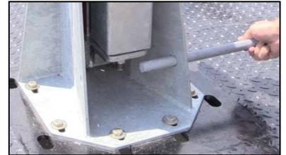
3. Use the lower hand winch to fold the mast down. Rotate the winch counter-clockwise until there is no more tension on the cable and the mast is set in its holder.
