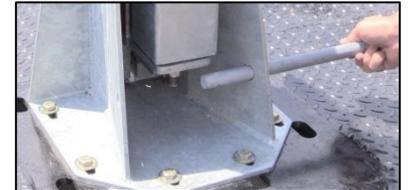
10. **Mast must be level!** Use a bubble level to level the mast before extending! Adjust outriggers until mast is level on all sides.
